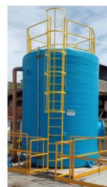
Figure 2: equalization tank installed
